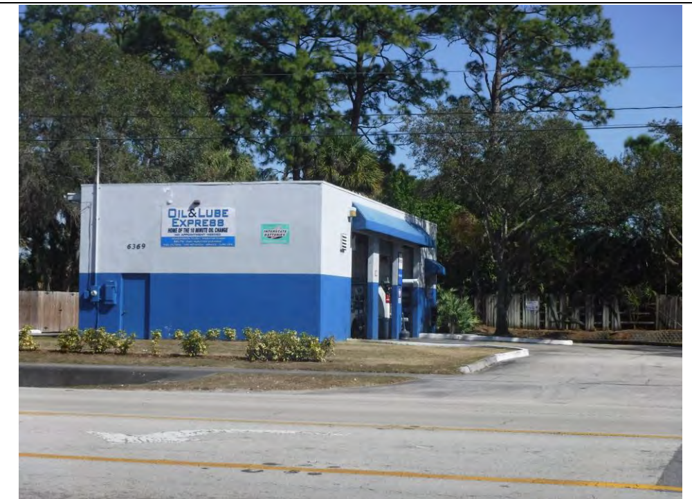
Photo taken from west of the property facing east. The Oil & Lube Center is visible.
