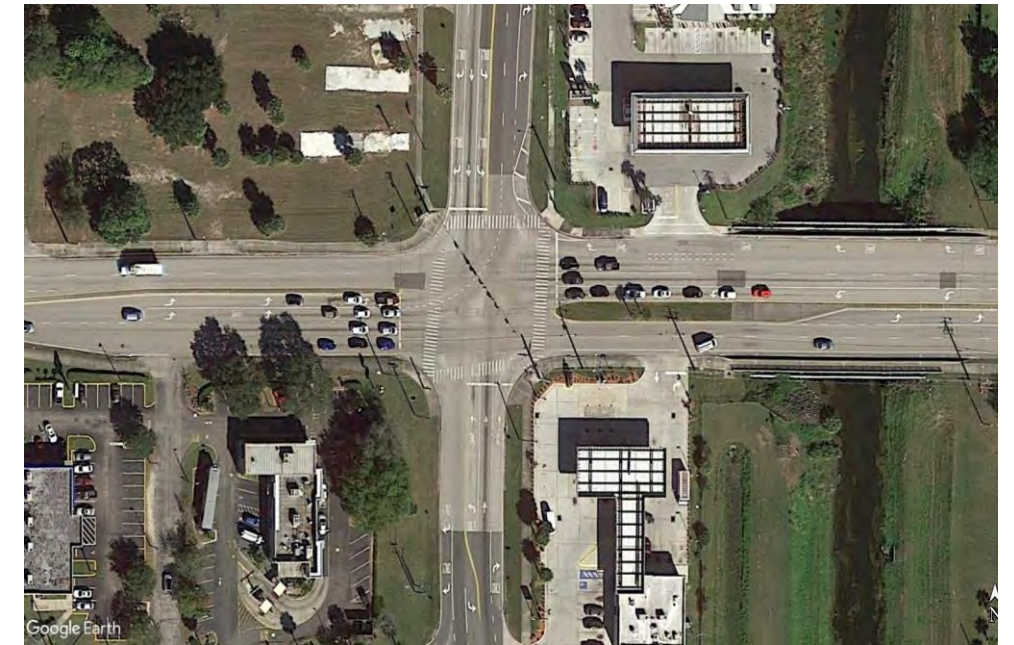
Photo taken from a 2020 aerial photograph showing the intersection of Malabar Road and Minton Road.
